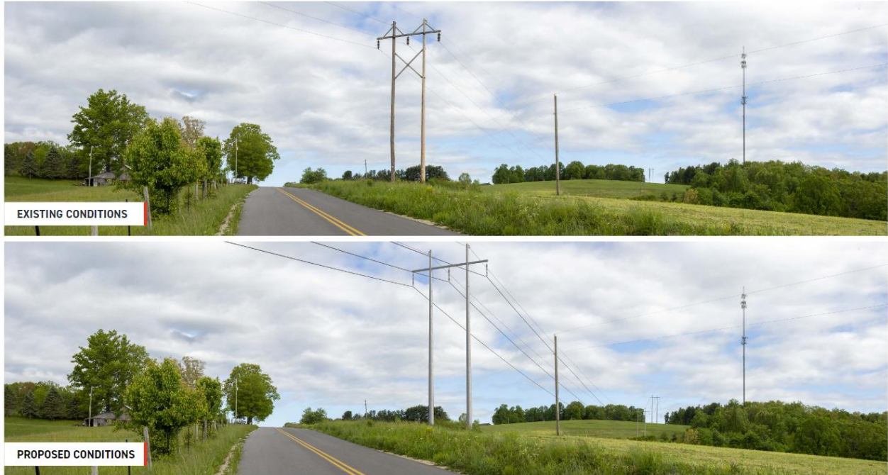
Figure 1. Comparable Existing and Proposed Single-Circuit H-Frame Structure (consisting of three conductors) Existing Wood H-frame (top) and Proposed Steel H-frame (bottom), which is the primary proposed structure to be used
