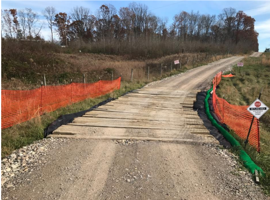
Figure 3. Temporary Access Road Construction
