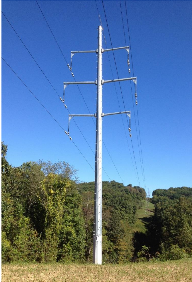
Figure 2. Comparable Steel Double-Circuit Monopole Structure (consisting of six conductors)
