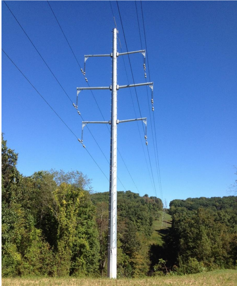
Figure 2. Comparable Steel Double-Circuit Monopole Structure (consisting of six conductors)
