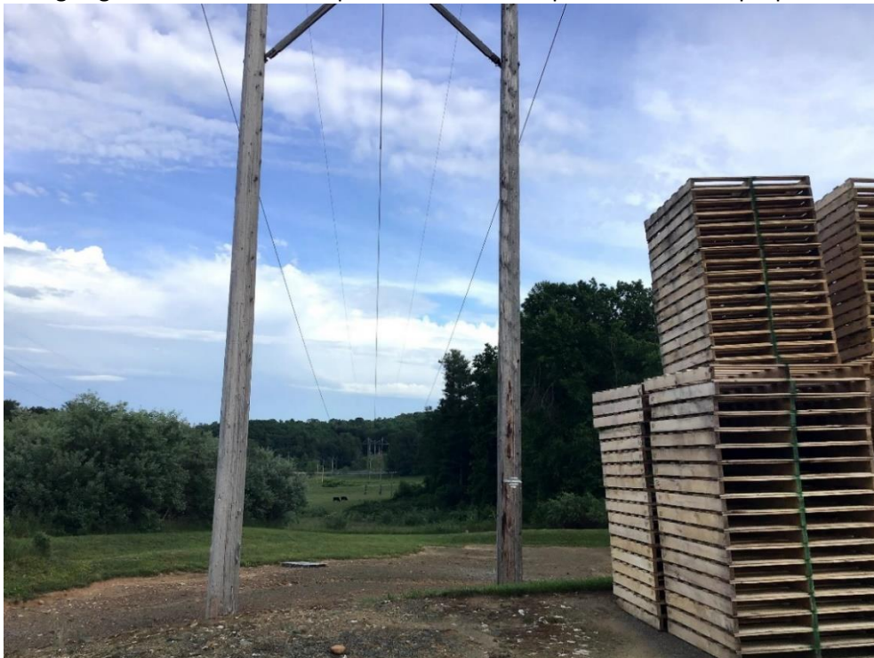
Photo 6. Existing ROW Exiting Floyd Substation
